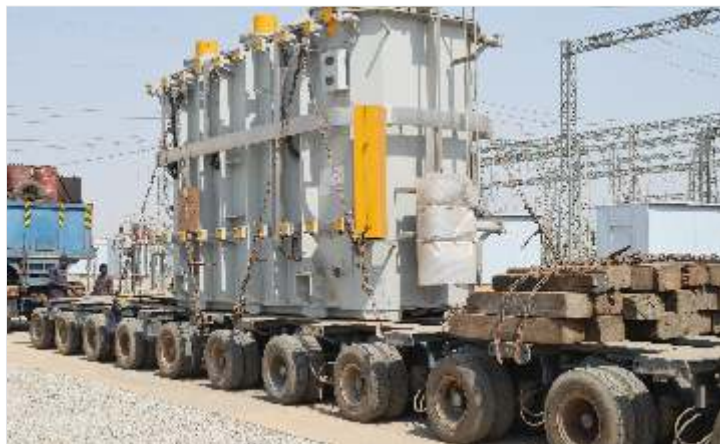
100MVA power transformer at 330/132/33kV Kumbotso Transmission Substation, Kano State.
