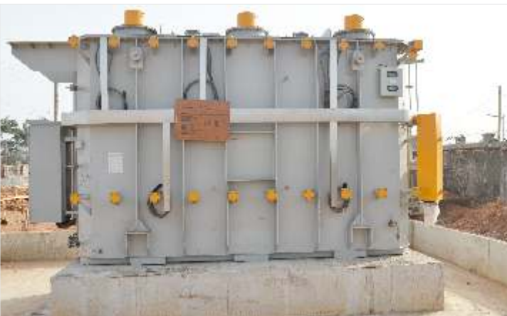
100MVA power transformer at Dan Agundi 132/33kV Transmission Substation
