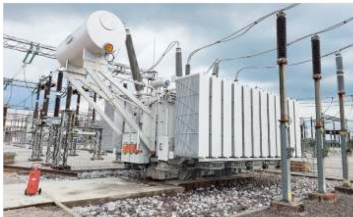
150MVA 330/132/33kV interbus transformer (IBTR) at Delta IV Transmission Substation, installed and energized
