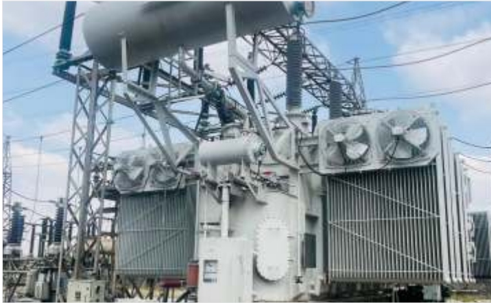
60MVA 132/33kV power transformer at Isolo 132/33kV Transmission Substation, installed and energised
