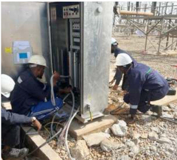
TCN engineers installing a brand new Circuit Breaker delivered to the Mando 330/132/33kV Substation, under the Kaduna Regional Office of TCN
