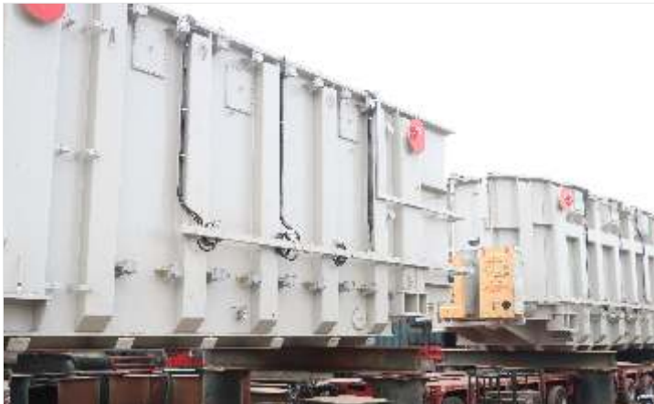
2x100/125MVA power transformers and accessories at Alagbon 330/132/33kV Transmission Substation.
