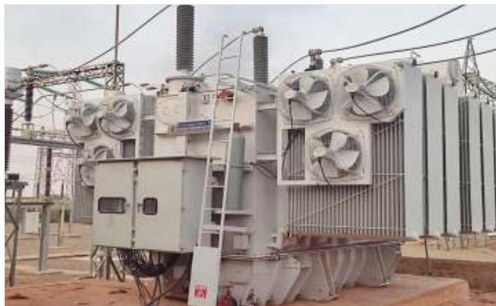
60MVA power transformer in Gombe 132/33kV Substation, installed & energised
