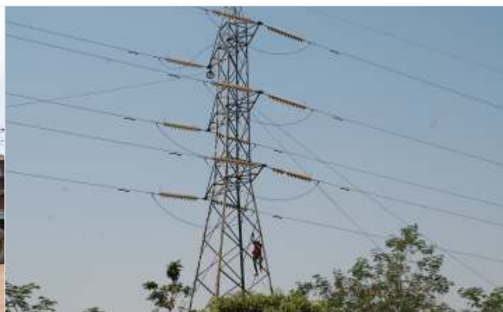
Ongoing reconductoring/upgrading of TCN Ayede-Eleyele 132kV Double Circuit transmission lines project in Ibadan.
