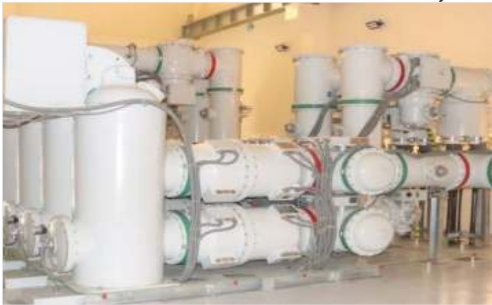
2X60MVA, 132/33kV Gas Insulated Substation (GIS) at Gwarinpa, Abuja
