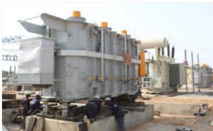
2x60MVA power transformers at 132/33kV Kankia Transmission Substation, Kastina State.
