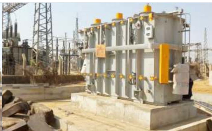
100MVA, 132/33kV power transformer at 132/33kV Dakata Substation, Kano, placed on plinth
